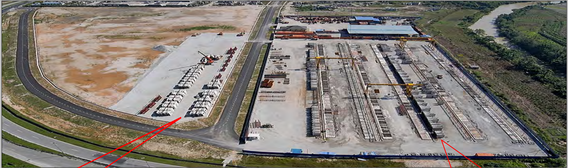
Proper storage yards
