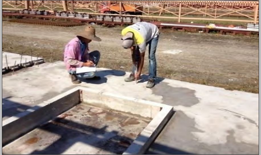
Rebound hammer test
