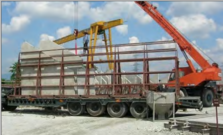
External transport to project
