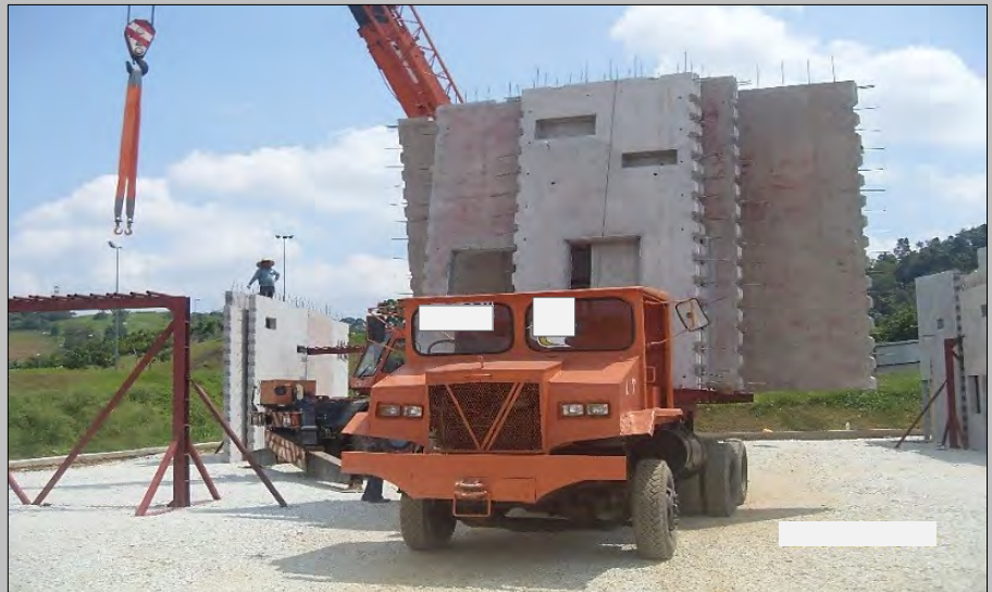
Internal transport to block yard
